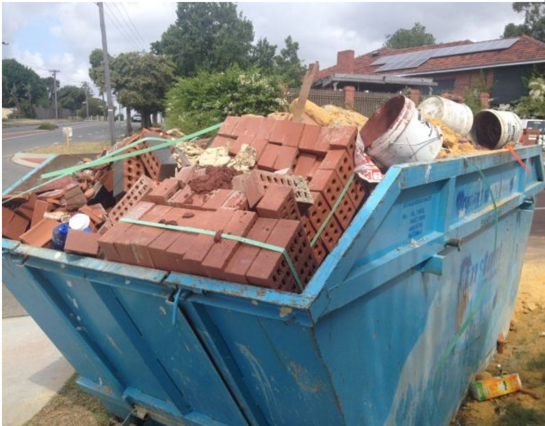
Figure 3. At least 3 leaves of strapped bricks dumped after small renovation in Floreat, WA. Not visible 20 steel rods 4m long and of 5mm diameter that were dumped. This is only what was visible.
