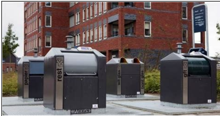
Fig 1-a : Various waste deposit containers in the Netherlands.
